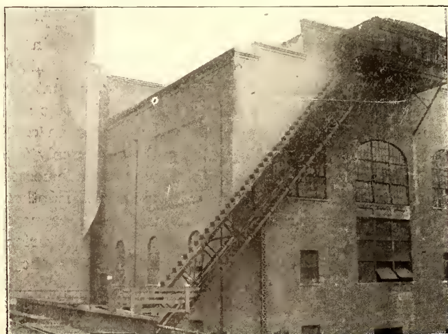
COAL AND ASHES HANDLING—CRUSHER AND BUCKET CONVEYOR, N. & W. RY. PLANT
